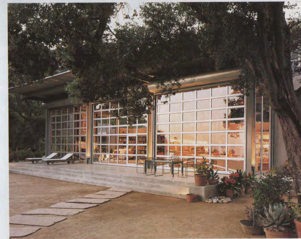
Lawrence Roll-Up Doors, Inc., L.A., also act as fireproofing. The table on the terrace is a modified Le Corbusier design.
