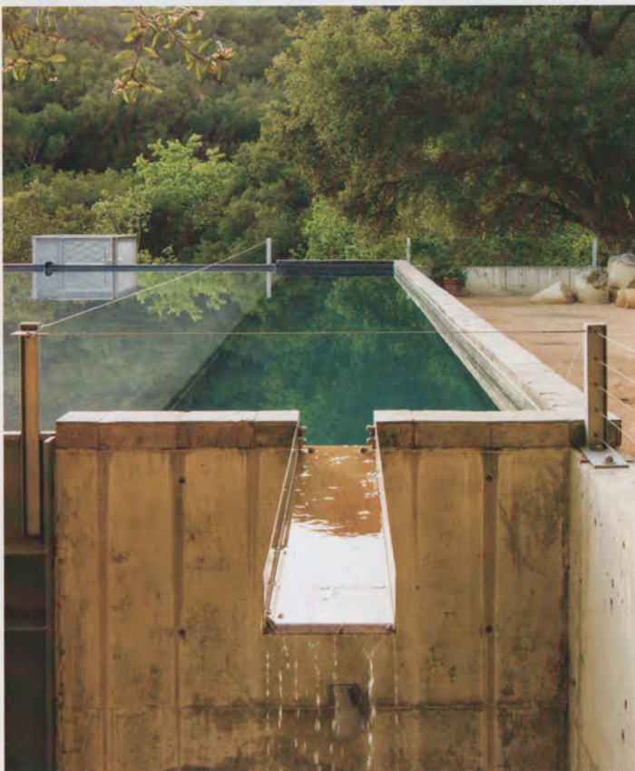
TOP, the garden and surrounding vegetation help stave off destruction from wildfires.
